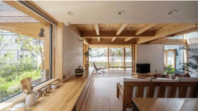
“Shisō-cedar house” : ecological building system for the Harima region (Hyogo Prefecture) Yamahiro wood builder Co., Ltd., Shisō-no-morinoki Co., Ltd. / Communication Yamahiro wood builder Co. uses the Shisō-cedar for approximately 90% of wood for the construction of this type of houses, and practically connects regional knowledge of the culture and environment of the Harima region. Yamahiro hopes that the Shisō-cedar house would develop a new landscape and promotes the exchange among residents in the city.
