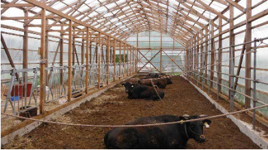
Roof Truss Unit for the Next Generation (Iwate Prefecture) Kiraku Souken Co., Ltd. / Technology and Research A brand-new roof truss unit using thinned wood. The volume of materials and the cost of processing can be reduced drastically. Since the number of components is limited, anyone can easily assemble the truss unit. This project would contribute to increasing use of thinned wood, and especially, lower-graded wood in the local primary industry.
