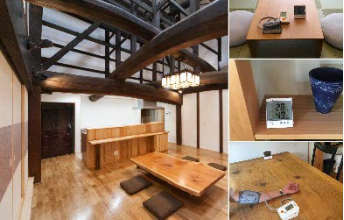
Renovation of Wooden Houses for Healthy and Comfortable Life (Aichi Prefecture) Shinwa Kensetsu Co., Ltd. / Technology and Research This project focuses on the thermal problem of wooden houses, which is the major driving factor for renovation. The project compared health conditions of residents and inside/outside temperatures of houses before and after the renovations, which evidenced health improvement of the residents.
