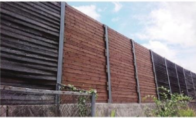
Wooden noise barrier (Nagano Prefecture) Nagano Prefecture Wood Sales Promotion Council /Wood Products Wooden noise barrier developed for the promotion of use in karamatsu (Japanese larch) of Nagano Prefecture.
